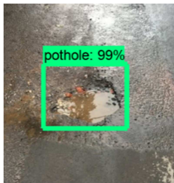
Figure 3.11: Detected pothole example.
