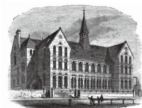
206.—JOHNSON STREET SCHOOL, STEPNEY.
