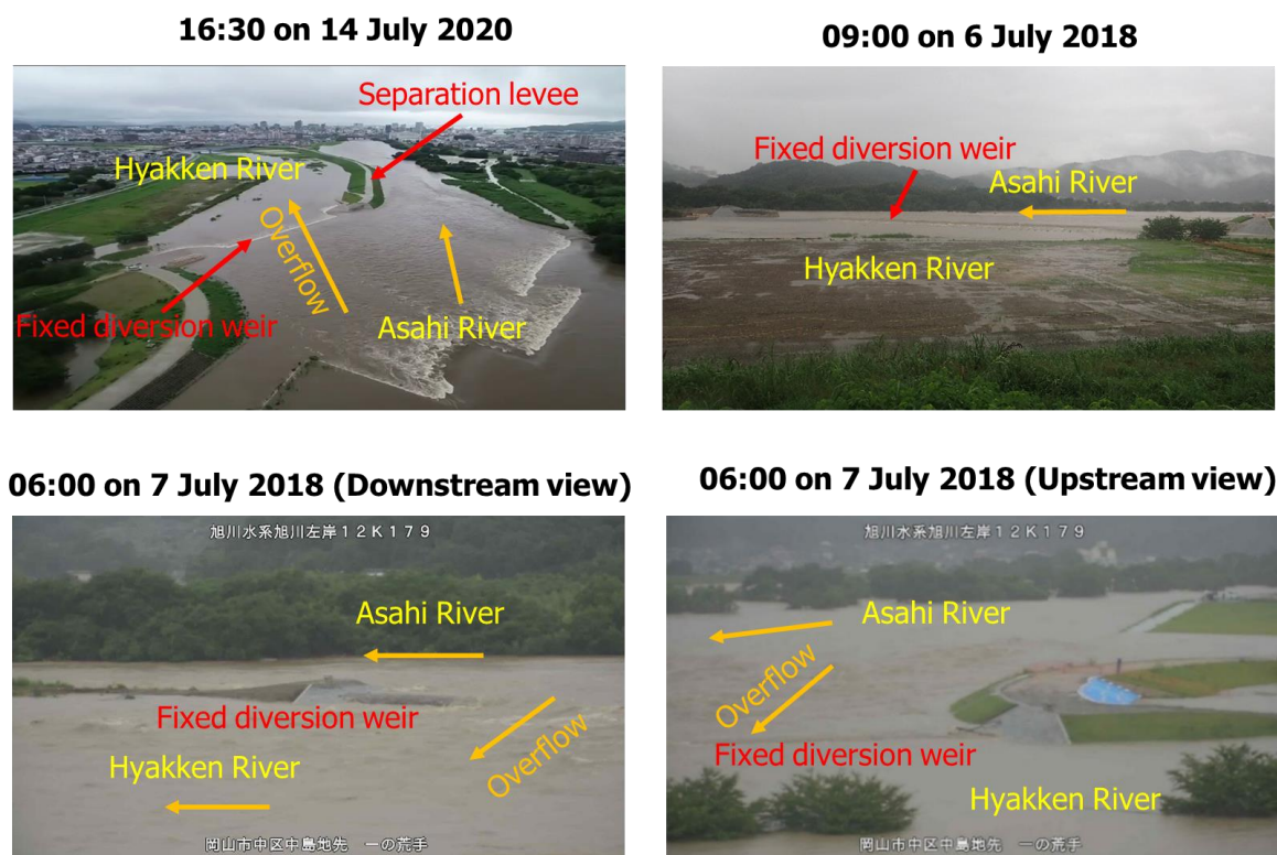
Figure 3.12 States of the diversion area during the 2020 and 2018 floods on the left bank of the Asahi River at about 12.2 KP.
