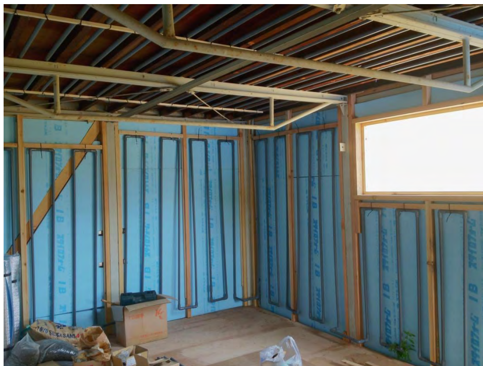
A 55—Piping network of the room at the study site on Tsushima campus, Okayama University (1).
