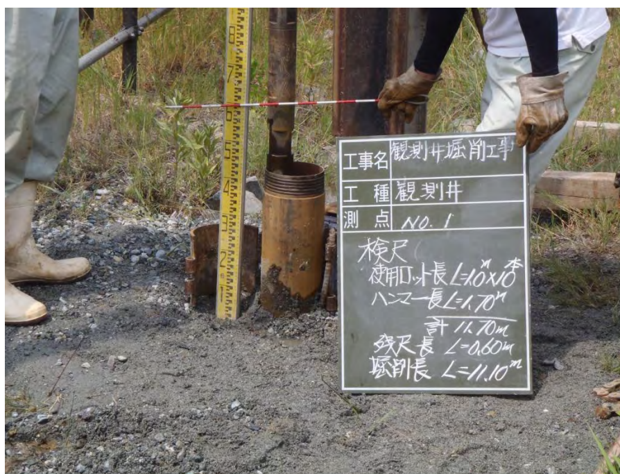
A 43—Installation of injection well No.1.
