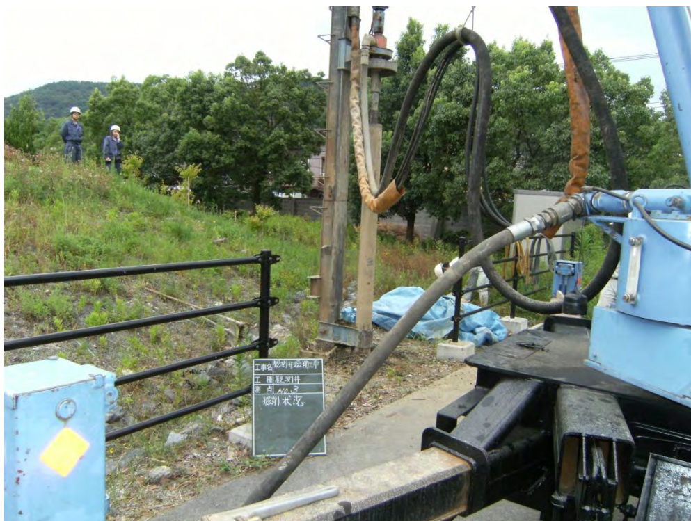
A 42—Installation of observation well No. 3’.
