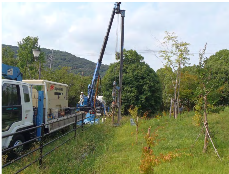
A 44—Installation of pumping well No.2.
