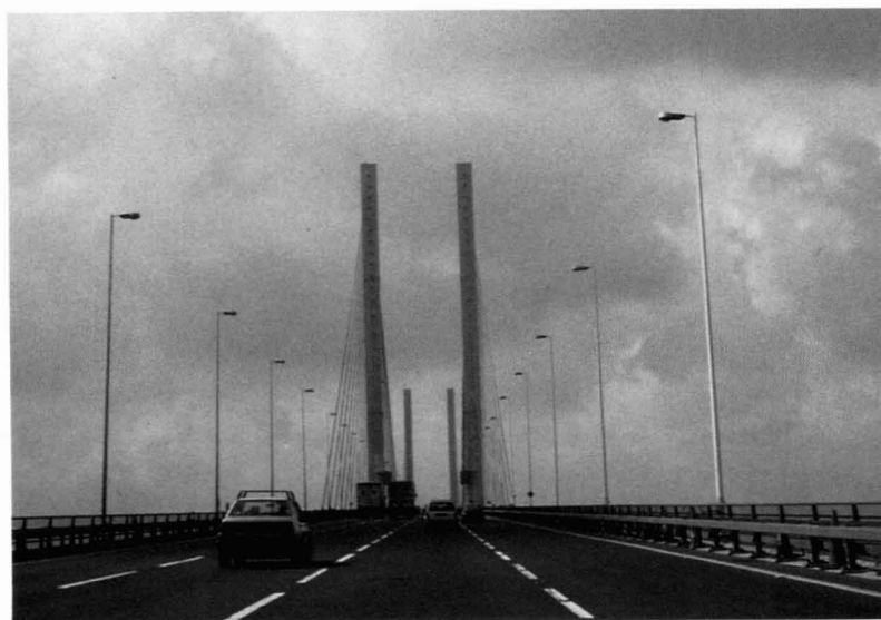
Photo 1. Queen Elizabeth II Bridge on M25
